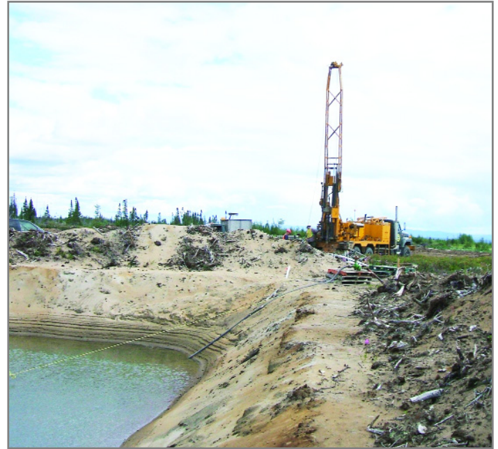
CBCL's sub contractor Logan Geo-Tec drills a monitor well along side of the experimental irrigation pond excavated by the owners of Grand River Farm.
